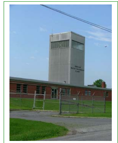
Oberlin Water Treatment Plant
