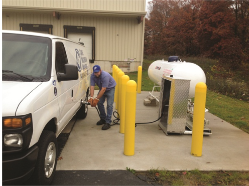
Figure 5: Example propane refueling infrastructure
