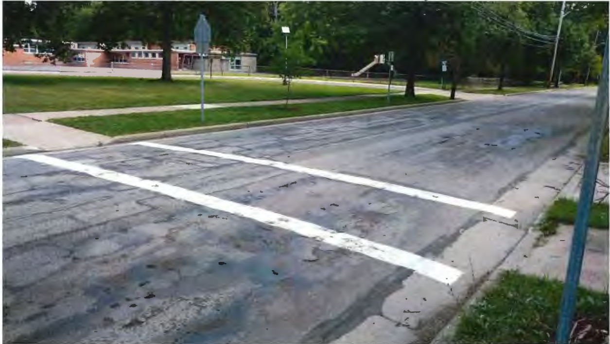
Non-compliant ramps at elementary school crosswalk. Typical pavement conditions.
