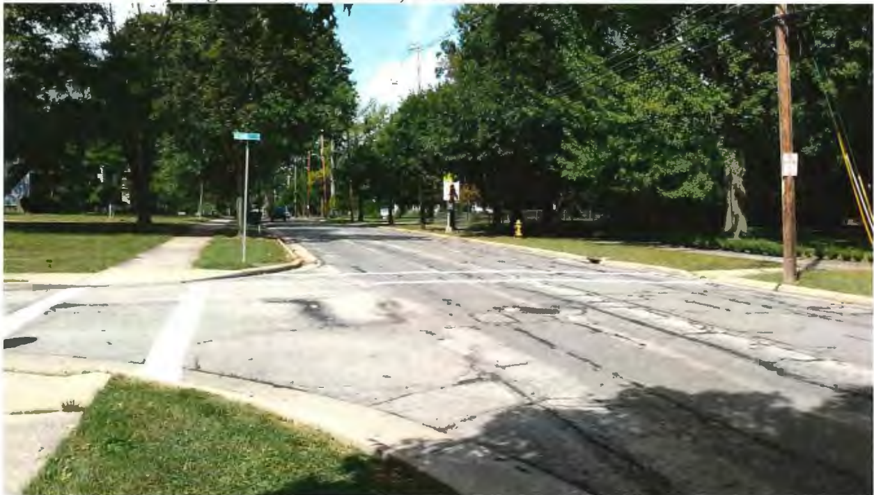
Non-compliant ramps at Spring Street Intersection. Typical pavement conditions.
