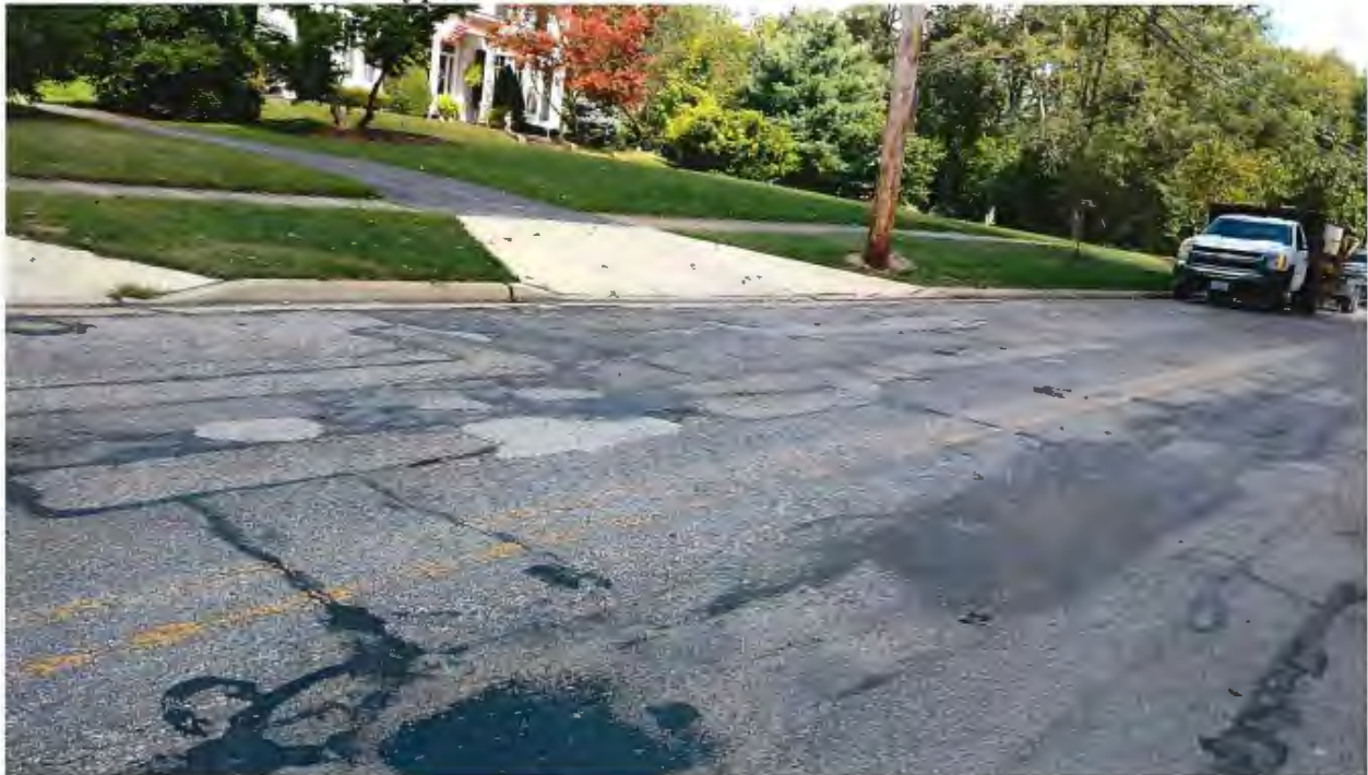
Typical pavement conditions: moderate rutting/distortion in travel paths; extensive block cracking; moderate raveling. Potholes forming.
