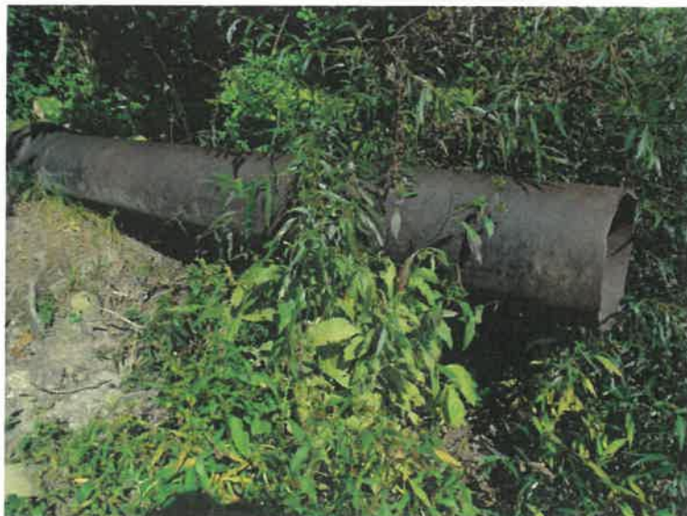
3. One of multiple unused piping located within the embankment.
