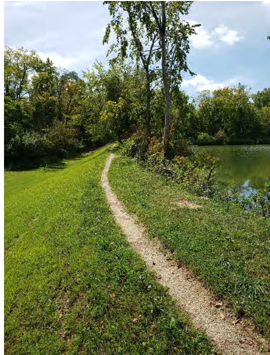
FIGURE 8 - EAST EMBANKMENT OF RESERVOIR NO. 1 WITH VEGETATION
