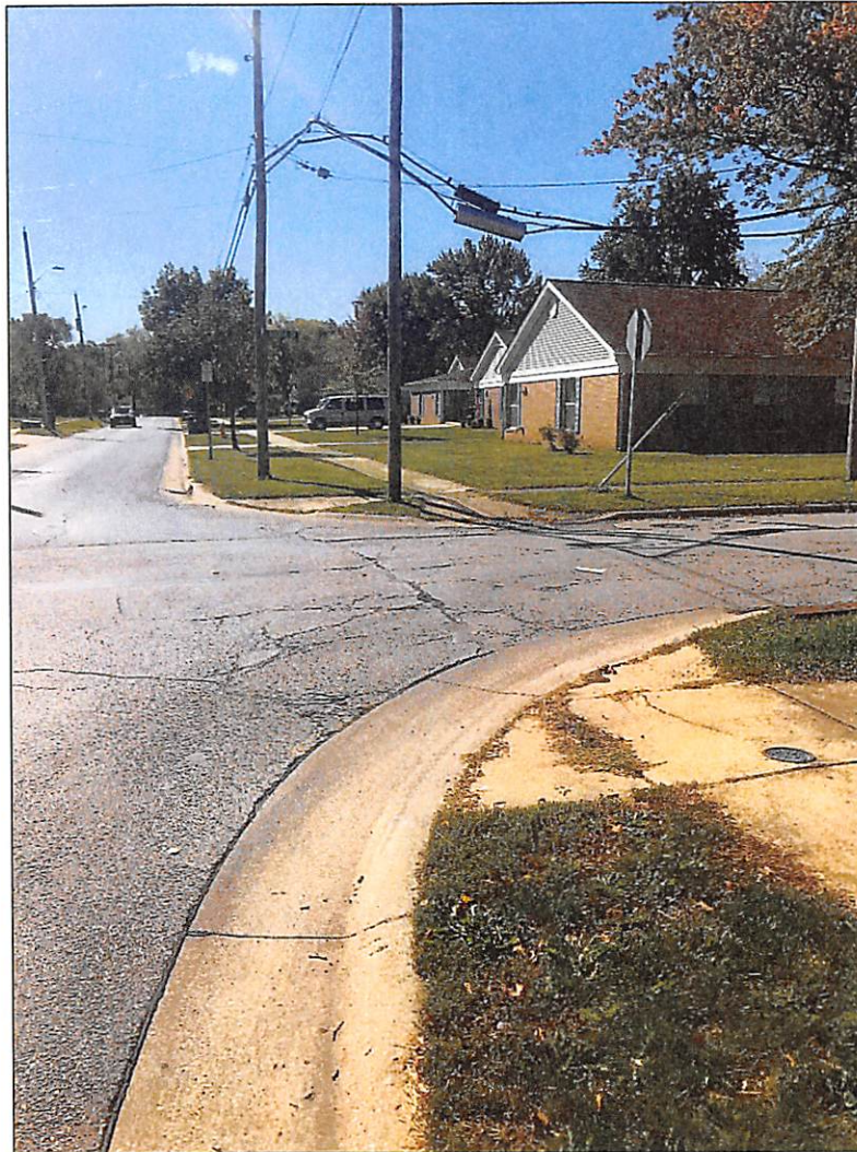
Unmarked crosswalk (typical all 3 legs). Non-compliant ramps. Typical pavement conditions.
