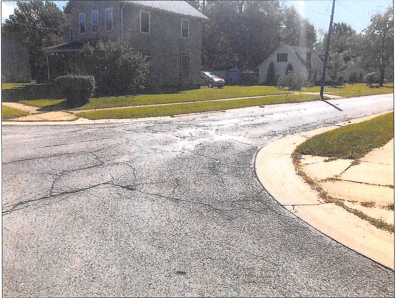
Unmarked crosswalk (typical all 4 legs). Non-compliant ramps. Typical pavement conditions.
