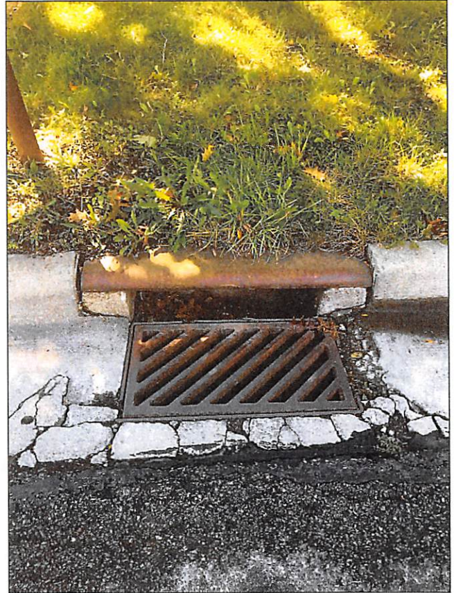
Severe cracking and pavement raveling
