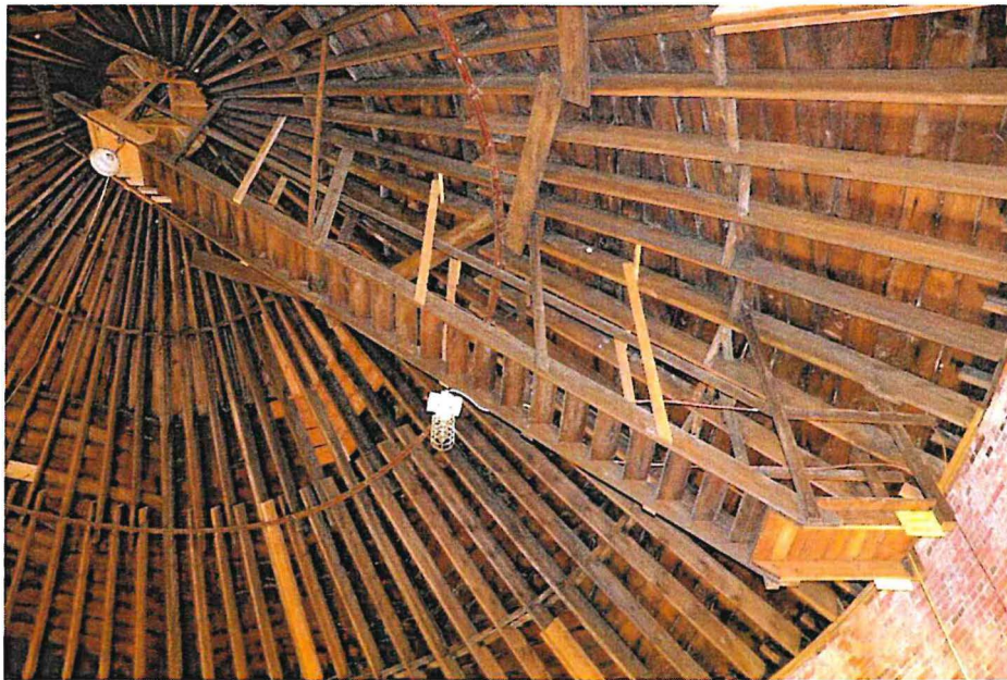
Photo 3. Staircase suspended from the Roof Structure
