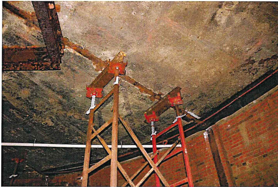
Photo 17. Temporary Shoring under the Embedded Beam
