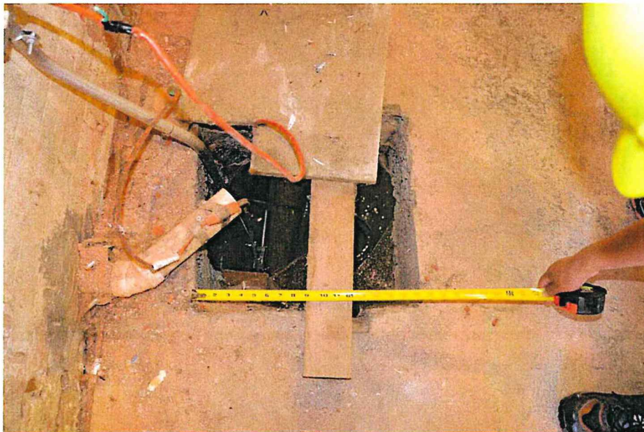
Photo 4. 18" X 18" Hole on the Main Floor
