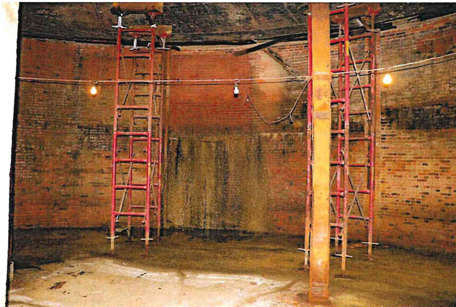
Photo 8. Active Leakage on the Basement Wall
