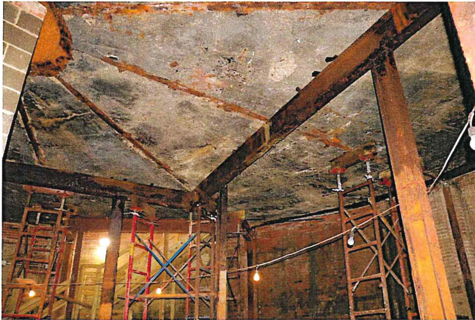
Photo 13. Main Support Frame in the Basement
