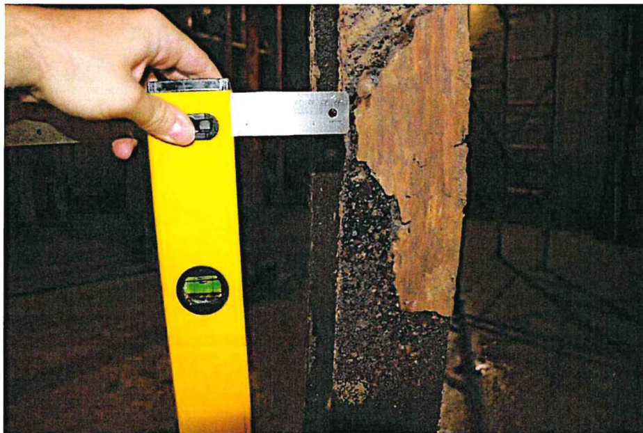
Photo 14. Column Buckled and Leaning
