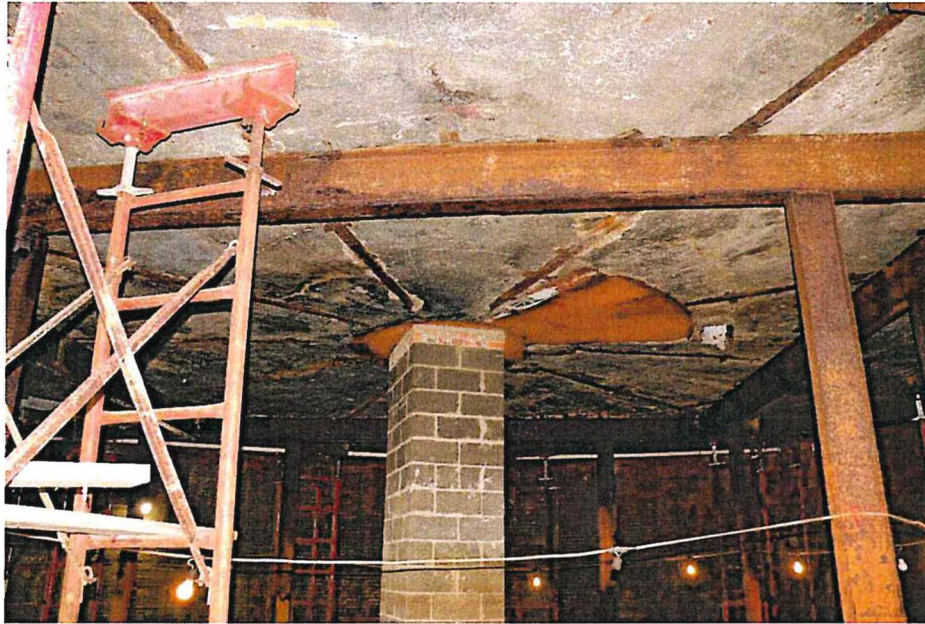
Photo 9. Center Masonry Column under the Main Floor
