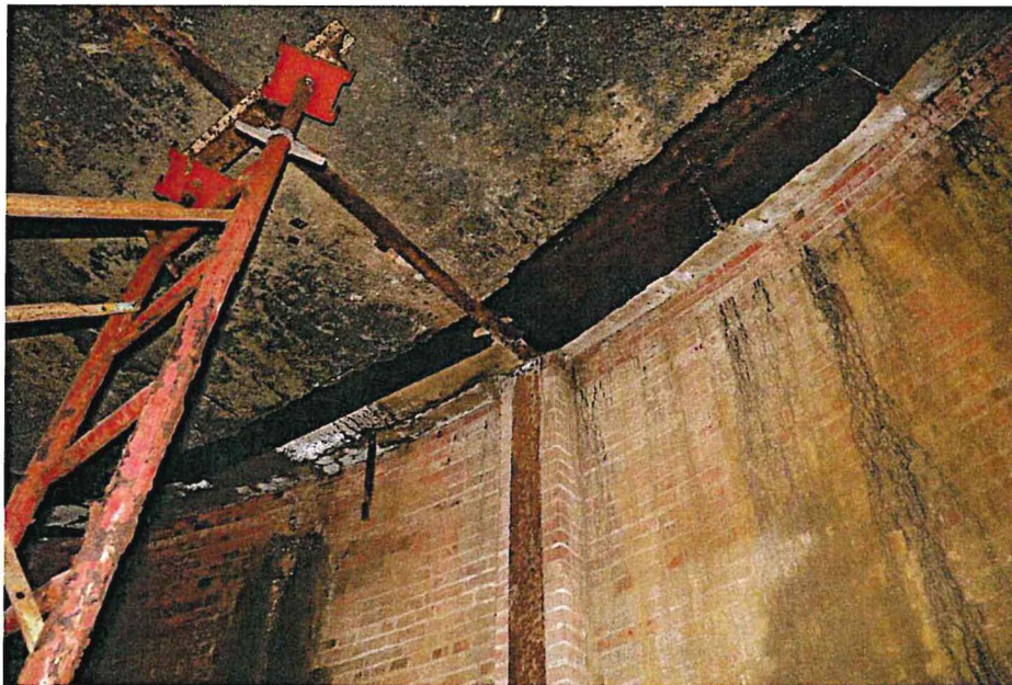
Photo 11. Embedded Beams and Columns in Basement
