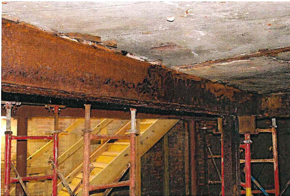
Photo 15. Main Frame Column with 100% Section Loss at Top
